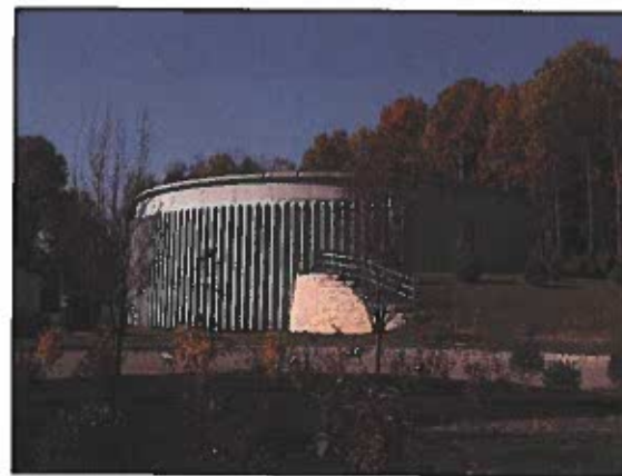
D115 Tank with Partial and Differential Backfill
