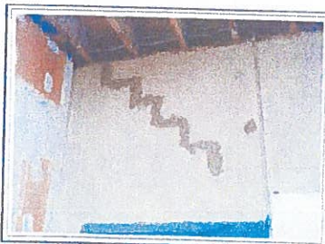
BAT REMEDIATION AREA IN FIRST GARAGE
